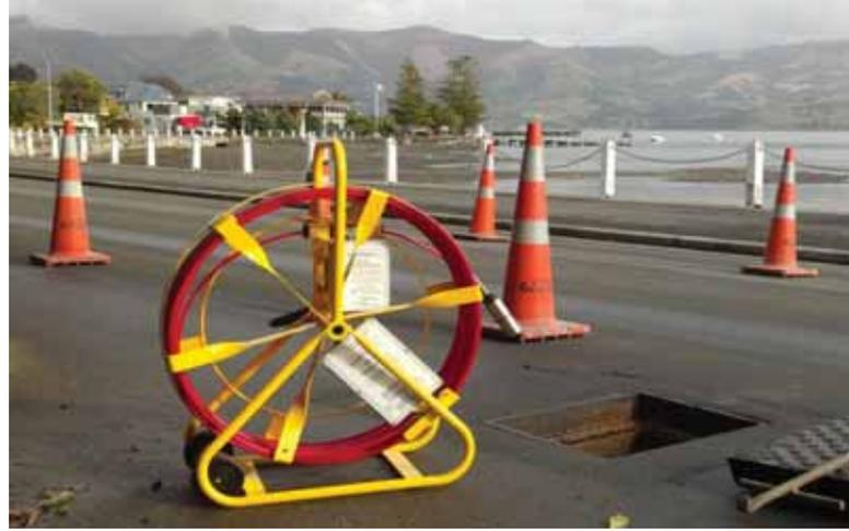
“A pipe which leaks water will also leak electricity, so when an Electro Scan user sends a current through a full non-metal pipe (for example brick, cement, reinforced concrete, plastic, pipe-lining resins, etc), they are able to measure the variation of electricity passing through the defects.”
