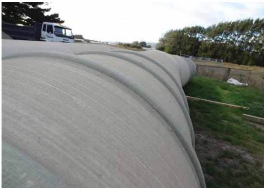
analysis. GRP ribs were also added to the bends to give added cohesion between the trench backfill and the geogrid thrust blocks. This provided extra safety against joint displacement due to thrust.
