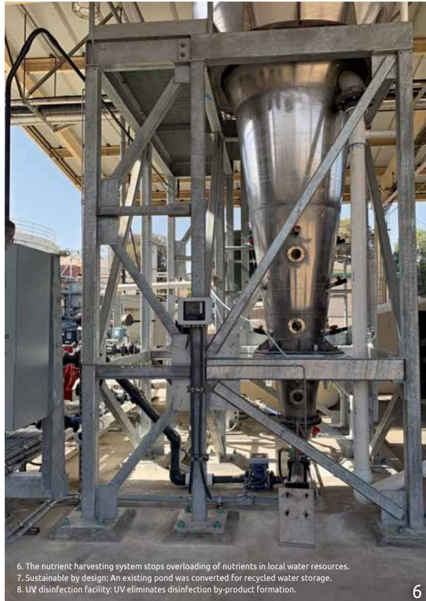
6. The nutrient harvesting system stops overloading of nutrients in local water resources.
