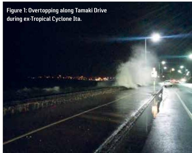
Figure 1: Overtopping along Tamaki Drive during ex-Tropical Cyclone Ita.
