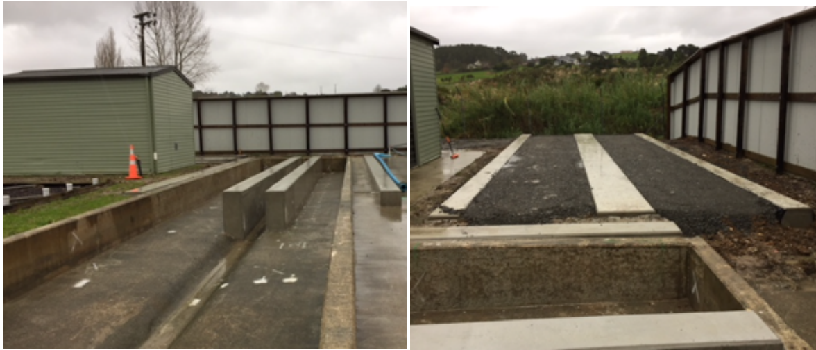
Figure 8 Strip footings for the two treatment plant trains at Warkworth
