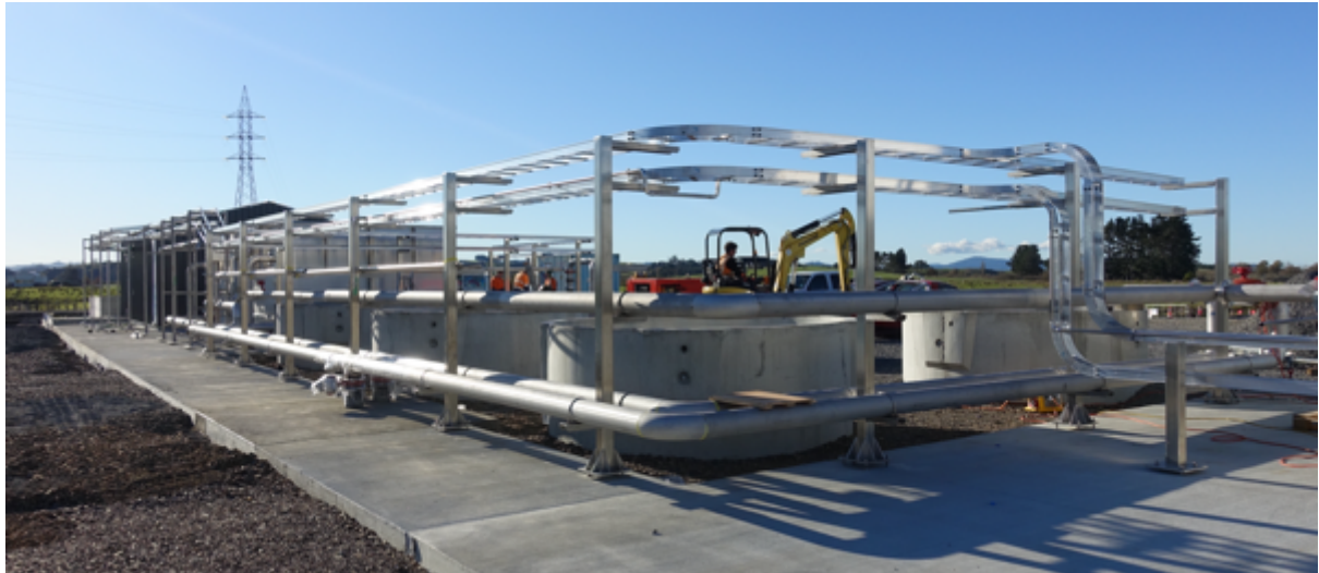
Figure 22 Meremere MBR Plant currently under construction
