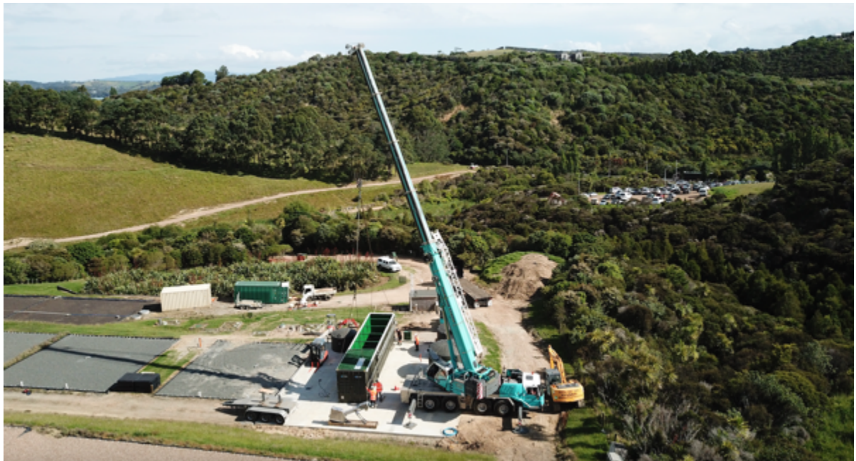
Figure 12 Container installation at the Owhanake site
