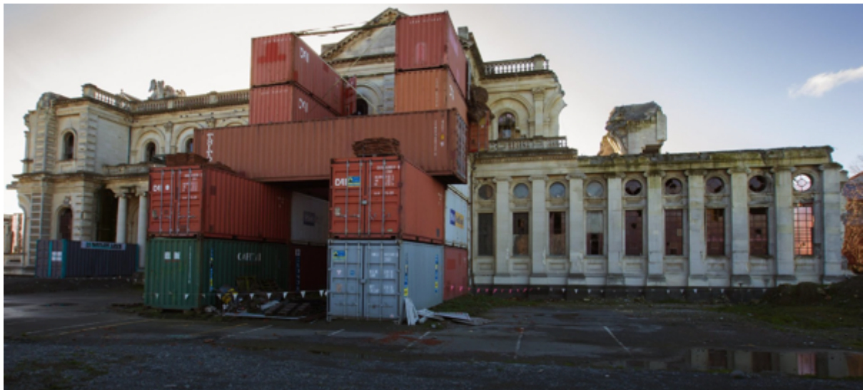
Figure 2: Shipping Containers prop up the Cathedral of the Blessed Sacrament, Christchurch [1]
