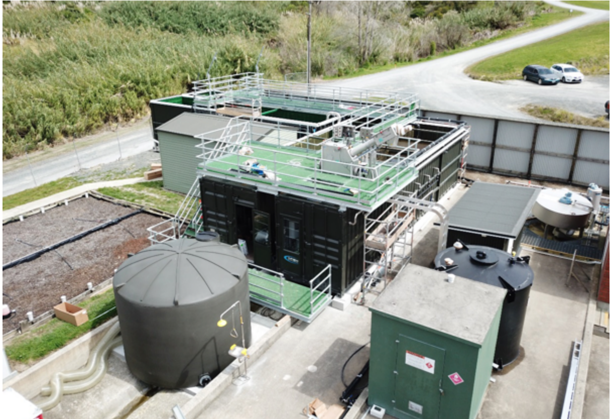
Figure 13 Completed Warkworth MBR plant wrapped around an existing site shed to make optimum use of limited space available
