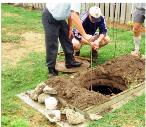
Checking scum and sludge levels in a septic tank
