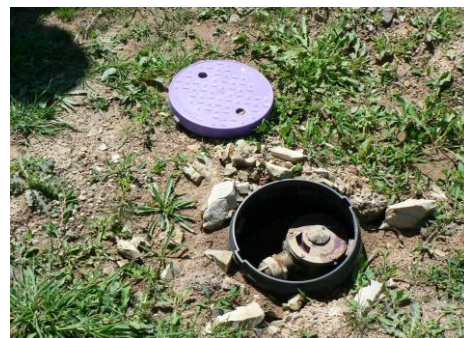
Automatic sequencing valve
