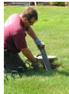
Lifting and hosing down effluent outlet filter
