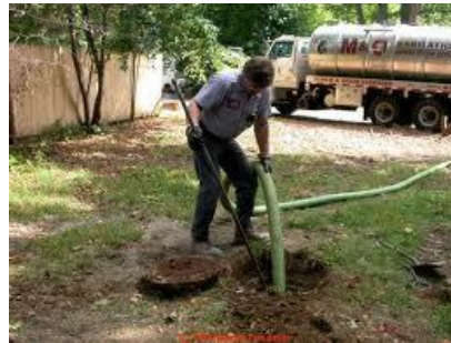
Septic tank pumpout
